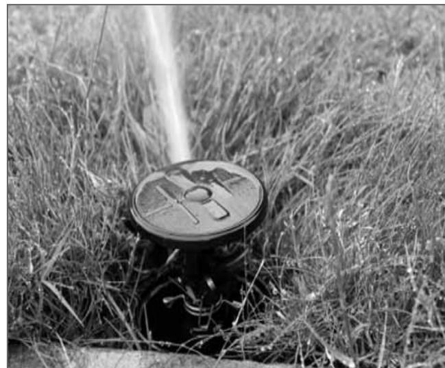
Underground irrigation systems also provide the potential for contamination. Much of the time after the lawn is watered, the sprinkler heads are submerged in puddles that could be contaminated with animal waste or fertilizers. If there is a loss of pressure in the household plumbing or the City distribution system, the contamination could be sucked back
